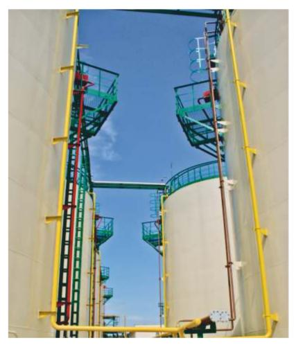
The storage section designated for high-melting oils is equipped with devices for heating and maintaining the storage temperatures to enable the product pumping.
